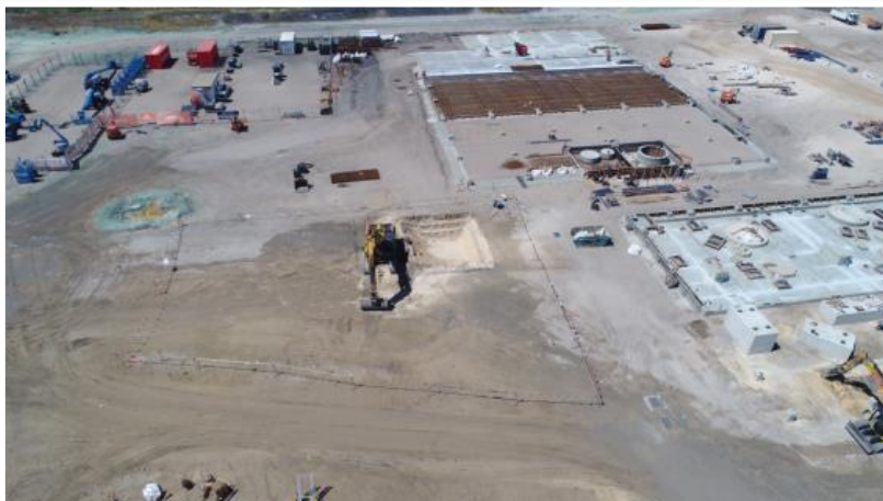
First excavation at the LHPP2 construction site
